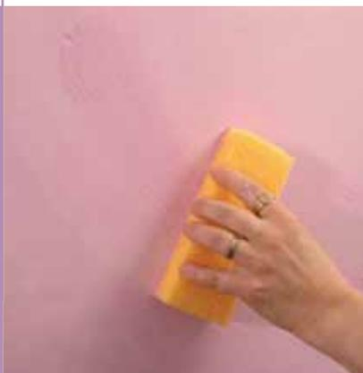
When you want a rougher structured surface, you can paint the wall surfaces first with Kevyt-Rae decorative coating. You can either apply the coating with a normal roller or make patterns on the rolled surface for example a spatula. On a structured surface, Taika Pearl Glaze should be applied with vertical brush-strokes from bottom up or with criss-cross. Further instructions can be found in the Tikkurila Pattern Painting Guide.
